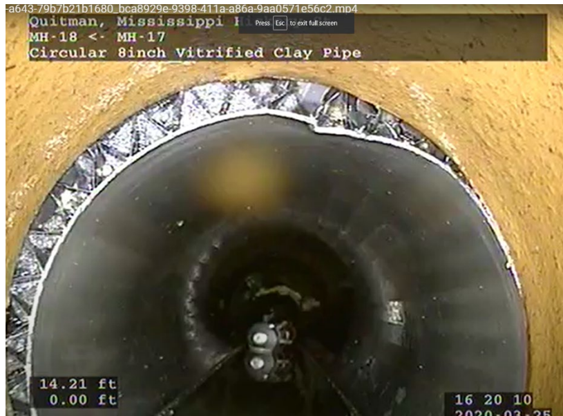
Figure 6 – Typical Joint Failure
