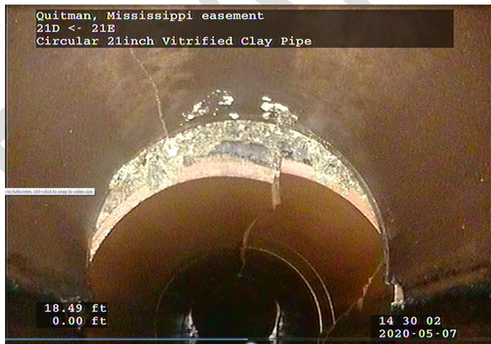
Figure 7- Typical Clay Pipe Failure
