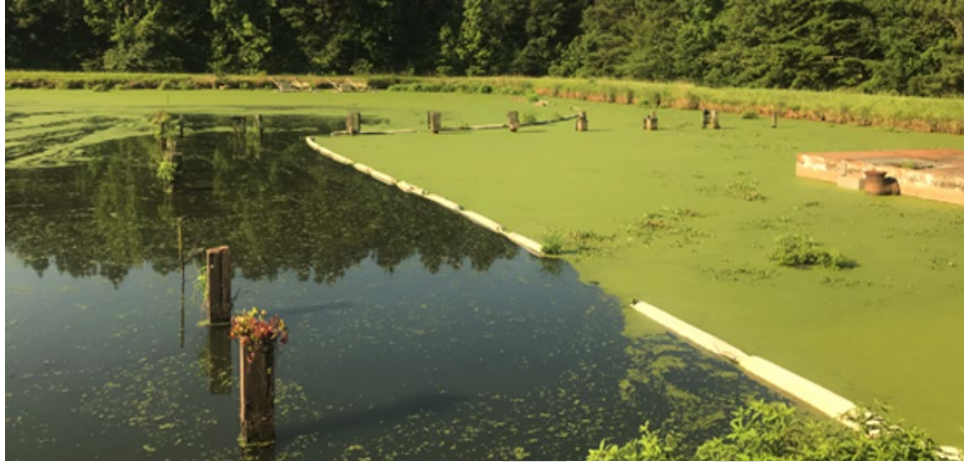
Figure 15 – Failed Baffle Curtain
